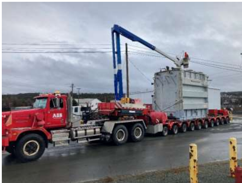
Figure 3: Spare Transformer Being Relocated
